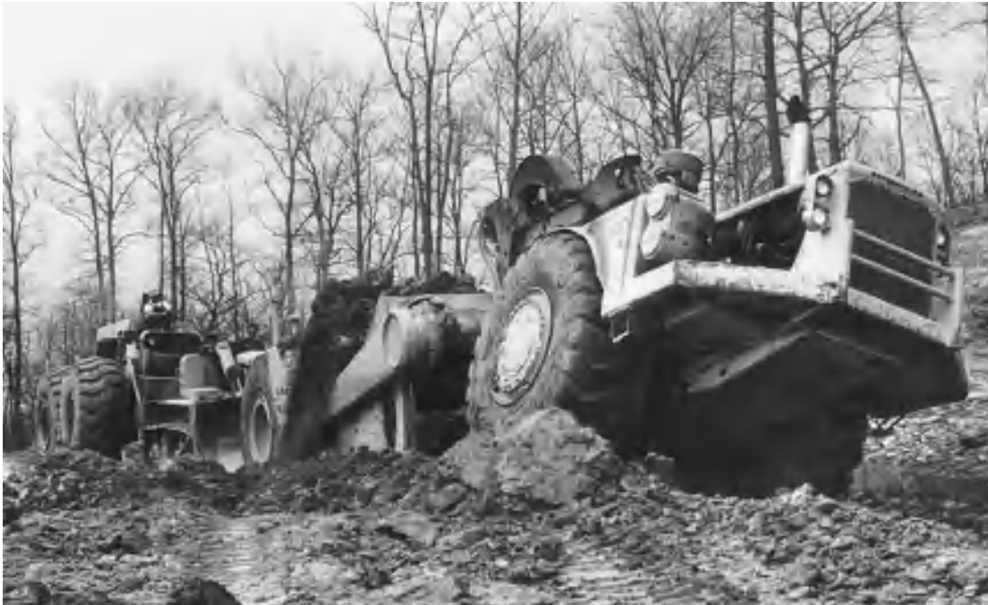
Fig. 5. A scraper in operation, as it is pulled by a tractor.
