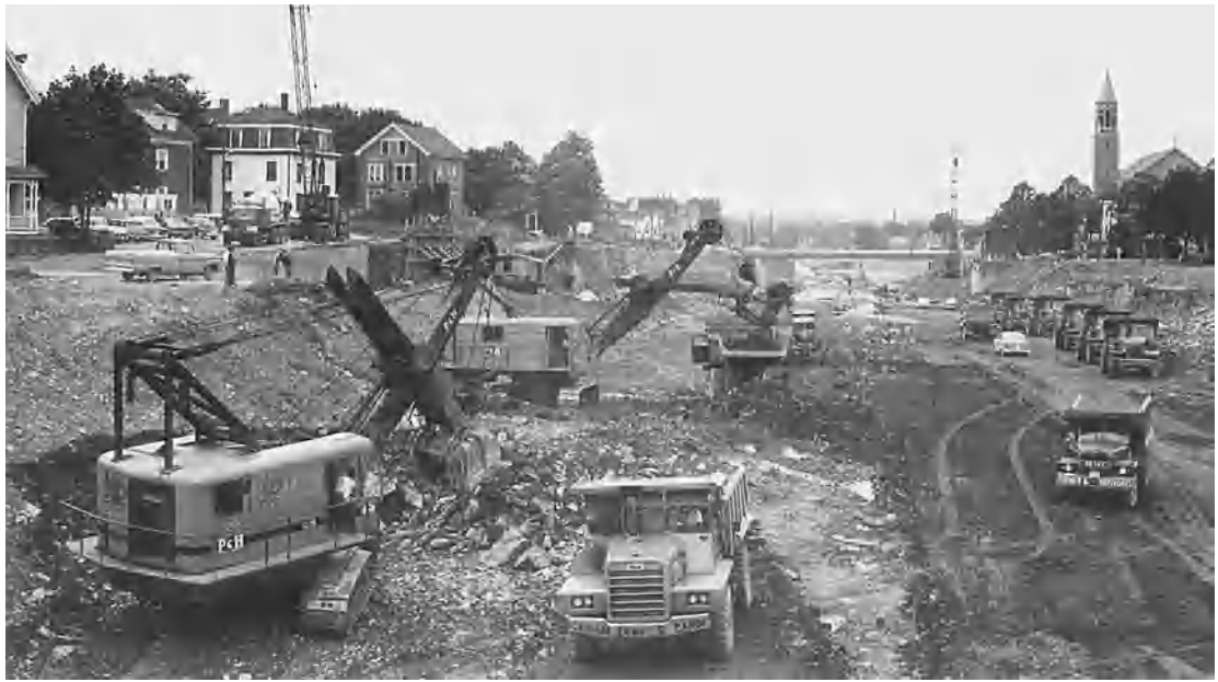
Fig. 3. Power shovels loading over-the-road rear-dump trucks.
