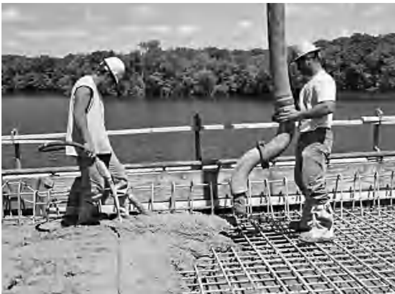
Fig. 1. Workers placing and vibrating concrete on a bridge deck including epoxy-coated reinforcing steel. (Portland Cement Association)
