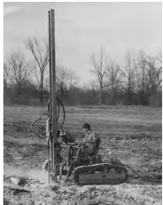
Fig. 7. Crawler-mounted drill. (Gardner-Denver)
