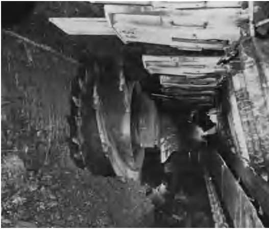
Fig. 16. Longwall shearer and hydraulic roof support.
