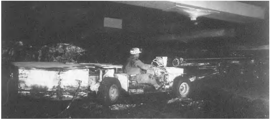
Fig. 10. Single-boom face drill operating in low-seam coal. (Long-Airdox Co.)
