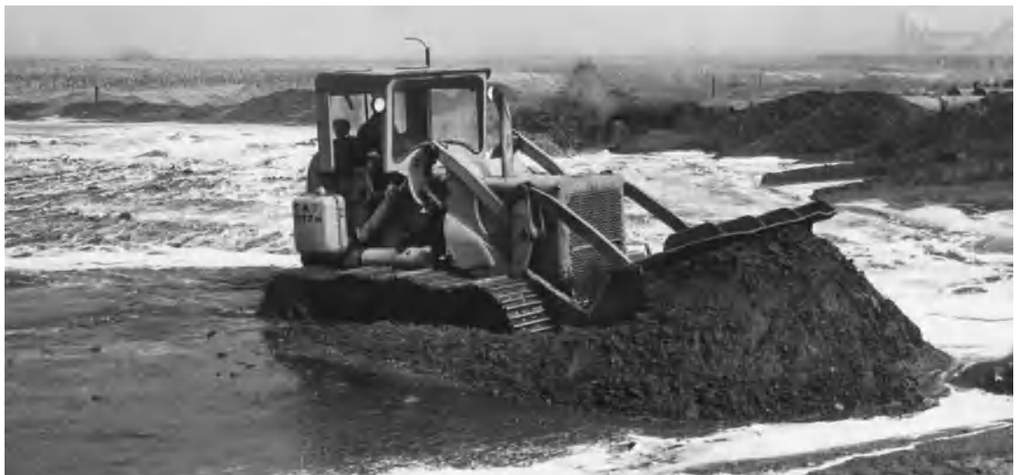
Fig. 4. A loader operating in a swamp.
