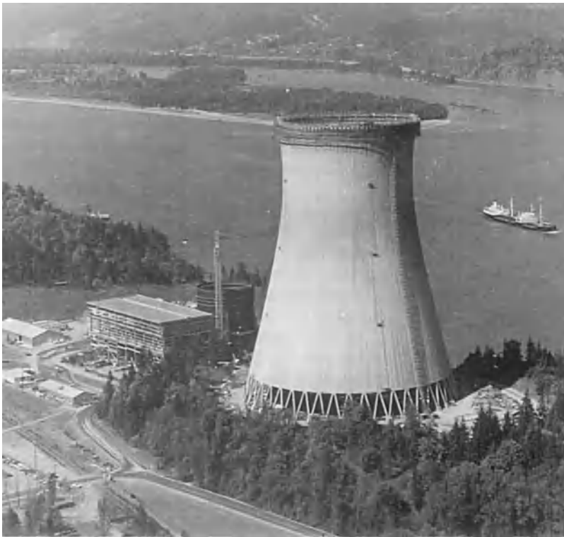
Fig. 1. Counterflow natural-draft cooling tower at Trojan Power Plant in Spokane, Washington. (Research-Cottrell)
