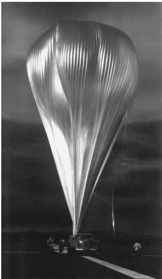
Fig. 1. Inflation of zero-pressure balloon. (NASA)
