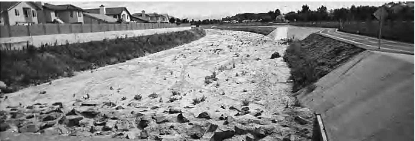
Fig. 2. Channelization of the Santa Gertrudis Creek in California showing bank protection and grade control structure traversing the channel bed.
