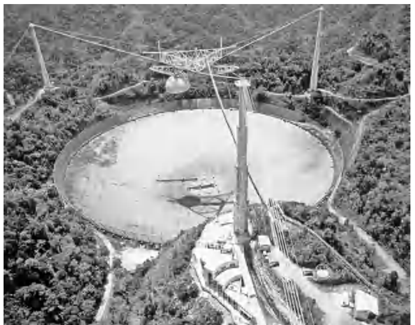
Fig. 2. The 1000-ft (305-m) NAIC fixed spherical dish near Arecibo, Puerto Rico. (NAIC/NSF-Arecibo Observatory)
