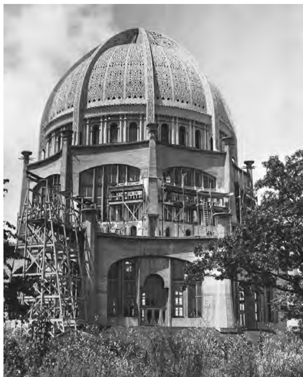
Located in the Chicago suburb of Wilmette, Illinois, this Bahá'í house of worship is the only temple of its kind in the United States. The building and lacelike dome of concrete and glass are nine sided. © HULTON-DEUTSCH COLLECTION/CORBIS.
