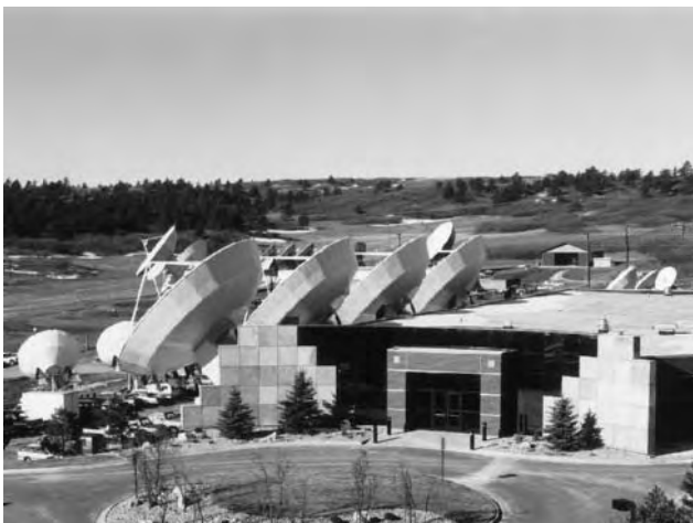
Figure 2. This DTH site in Colorado uses four 13-m antennas for uplink operations and numerous smaller dishes for programming reception. Courtesy of DirecTV, Inc.
