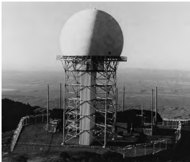
Figure 21. The ARSR-4 is a long-range, three-dimensional, solid-state surveillance system. It was specifically designed as a joint-use radar for the FAA, the U.S. Air Force, and US Navy. The ARSR-4 detects all aircraft out to 463 km through all weather and clutter conditions as well as man-made interference. (Photo courtesy of Northrop Grumman Corporation.)
