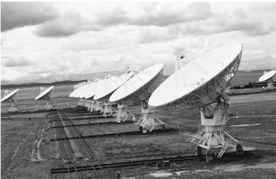
Figure 2. The Very Large Array (VLA) in New Mexico is a radiotelescope consisting of 27 shaped 25-m dual-reflector antennas. (Courtesy of the National Radio Astronomy Observatory—NRAO/AUI/NSF).
