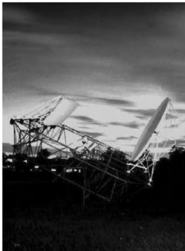
Figure 11. Photograph of a Cassegrain feed arrangement and parabolic reflectors.
