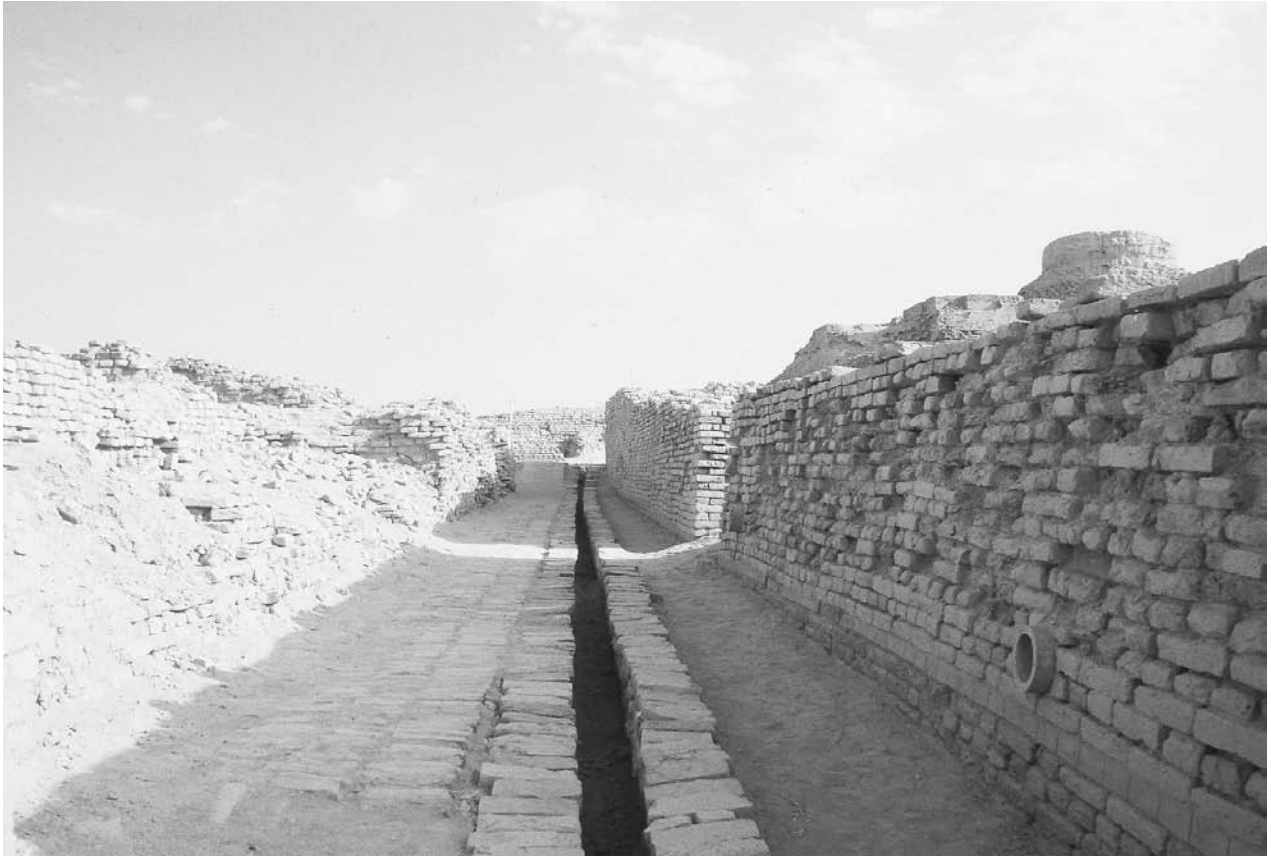
Brick Wall and Drain Excavated at Mohenjo-Daro. Due to the nature of the topography and the intensity of floods along the Indus and its tributaries, ancient settlements were not able to maintain major canals for irrigation, although they frequently constructed drains for redirecting floodwaters. FOTOMEDIA ARCHIVE.
