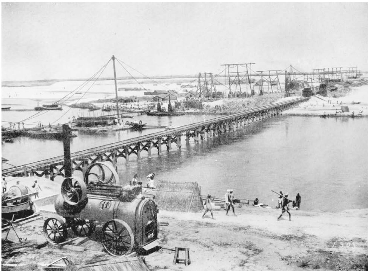
Curzon Ganges Bridge, Allahabad. Under Lord Curzon's rule as viceroy, the Raj initiated the development of an extensive rail and bridge network throughout India, partly to stimulate trade, partly to facilitate troop movements. The result was that by 1910 India had the fourth-largest railway system in the world. SURVEY OF INDIA / AKHIL BAKSHI.
