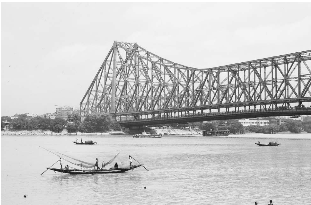
Gateway to Kolkata. The imposing Howrah Bridge over the Hooghly River (a tributary of the Ganges, where all life is said to begin). It is one of the finest examples of a cantilever bridge. AMIT PASRICHA.
