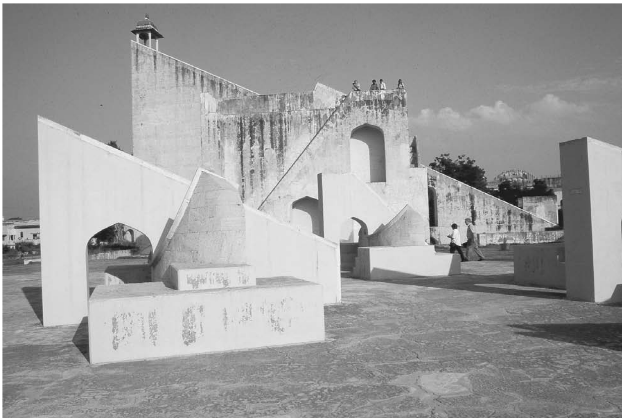
Observatory in Jaipur. In Jaipur, one of five Jantar Mantar (literally “instrument for calculation of the heavens”) constructed at the behest of Maharajah Sawai Jai Singh II between 1727 and 1734. These national observatories incorporate multiple buildings of unique form (each with a specialized function for astronomical measurement), monumental scale, and lavish materials. ADITYA PATANKAR / FOTOMEDIA.
