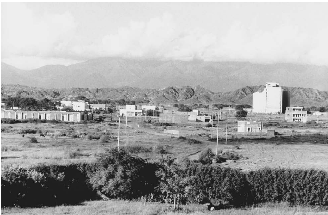
Secretariat Building in Chandigarh. To the right, the Secretariat, one of a series of government buildings on the northern fringe of Chandigarh designed by Le Corbusier, the French modernist architect, in the 1950s. The buildings' monumental size and scale were consonant with both the aspirations of Prime Minister Nehru who was eager for symbols of greatness for the new capital, and the splendid Himalayan landscape in which they are set. TIME LIFE PICTURES/GETTY IMAGES.
