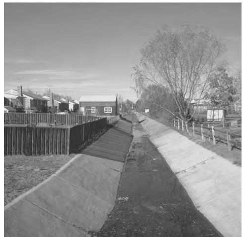
Plate 131 Concrete-lined channels and restrictive boundary conditions complicate urban stream restorations
