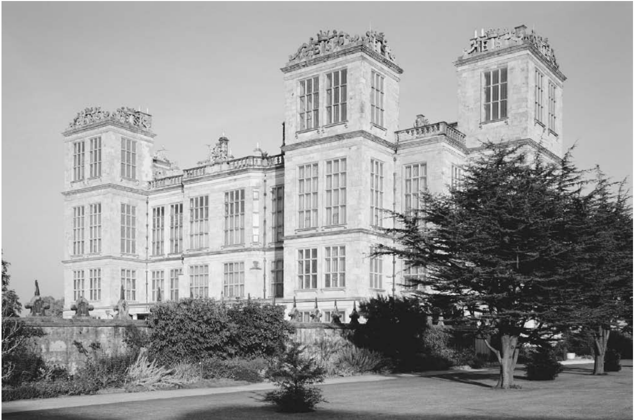
Exterior of Hardwick Hall near Chesterfield, England. © ERIC CRICHTON/CORBIS.
