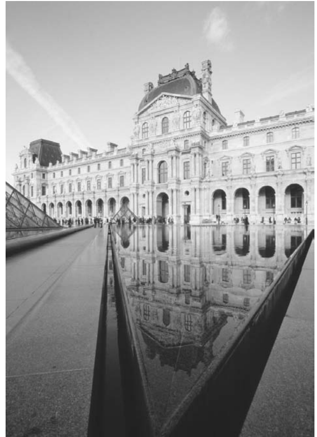
Façade of the Palace of the Louvre in Paris. © PHILIP GOULD/CORBIS.
