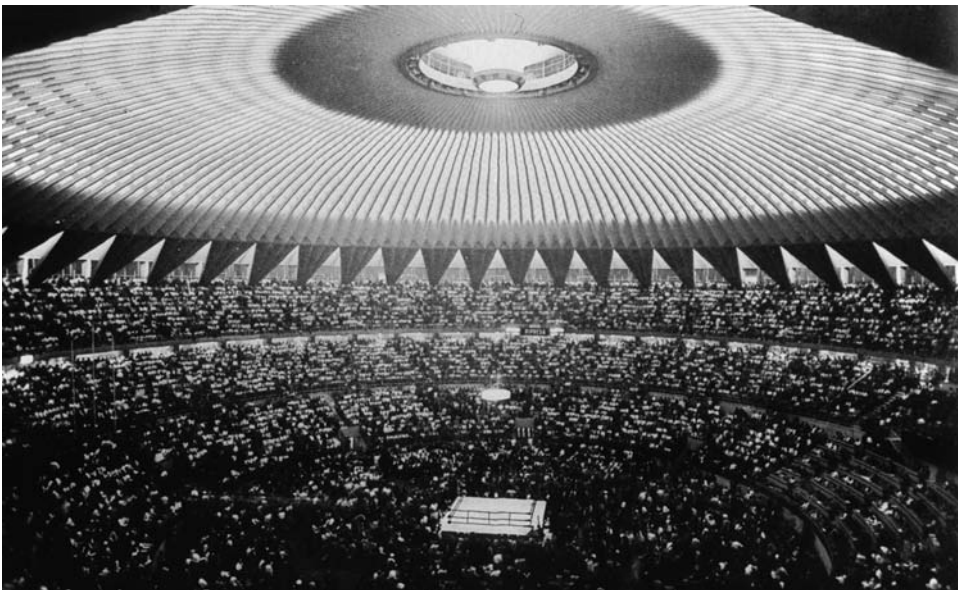
Figure 16. Sports hall for Olympic Games, Rome (1958) by Luigi Nervi. [Photo: Cement and Concrete Association.]
