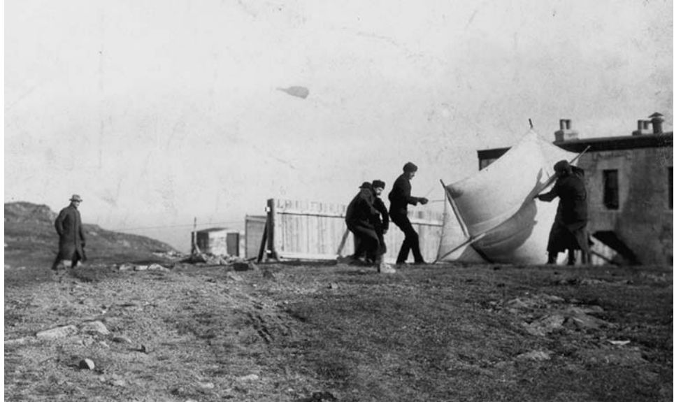
Figure 5. Marconi and his assistants launching the kite-supported aerial at Signal Hill, St. John's, Newfoundland, December 1901. [Courtesy of the Marconi Corporation.]
