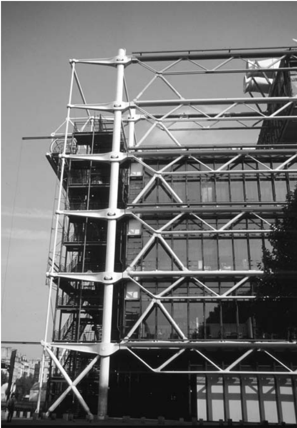
Figure 6. Pompidou Centre, Paris (1969–1974; engineered by Ove Arup and Partners). The exposed steelwork inside the building is fire-protected using intumescent paint. The main, vertical tubular columns are fire-protected by being filled with water, which would be pumped around to remove heat in a fire. [Photo: Bill Addis.]
