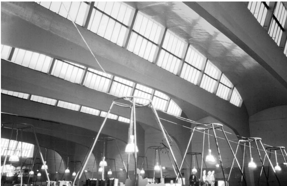
Figure 18. Market hall roof, Plymouth, by British Reinforced Concrete. [Photo: Bill Addis.]
