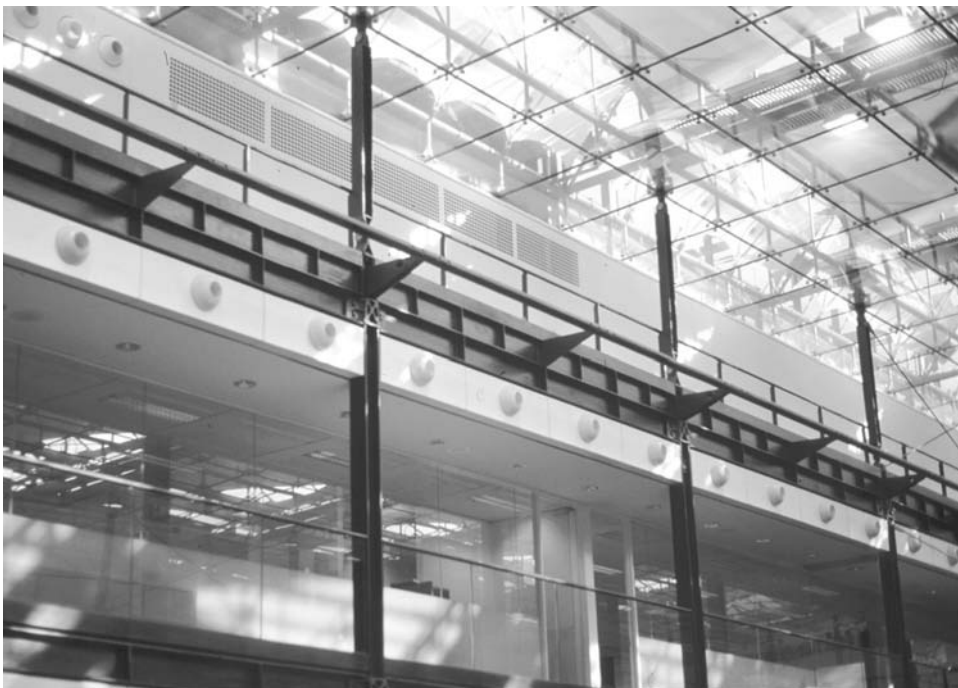
Figure 7. Bedfont Lakes near London (1993; engineered by Buro Happold). As a result of fire engineering design, none of the exposed steel needs fire protection.
