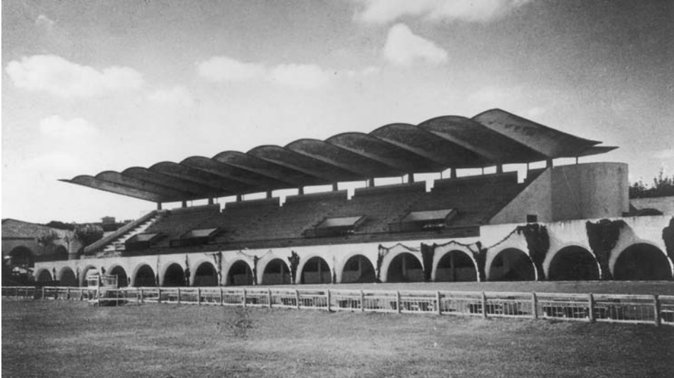
Figure 15. Stand at Madrid race course (1935) by Eduardo Torroja. [Photo: Cement and Concrete Association.]
