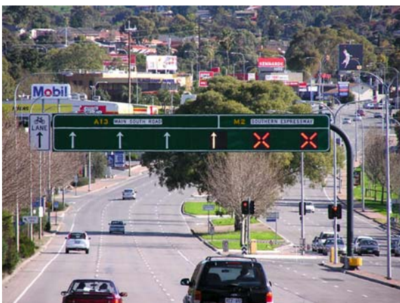
Contraflow in Transportation Network, Figure 8 Controlled access of automated reversible lane system in Adelaide (source: wikipedia.org)
