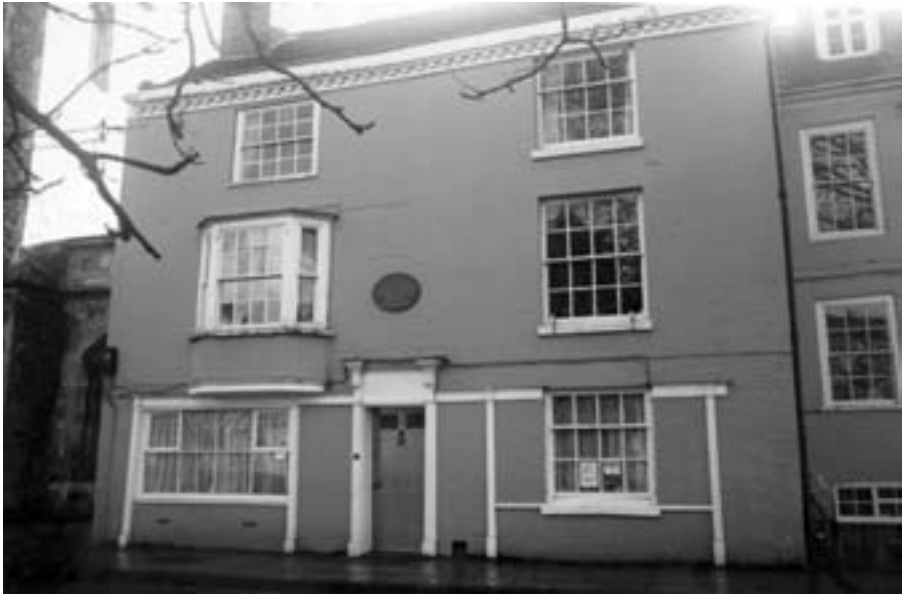
No. 8 College Street, Winchester, where Jane Austen died on 18 July 1817. She had been moved into lodgings here in May 1817 in order to receive better medical treatment.
