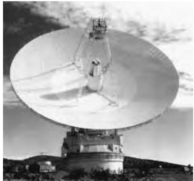
Front view of the 70-meter-diameter antenna at Goldstone, California. The Goldstone Deep Space Communications Complex, located in the Mojave Desert in California, is one of the three complexes that make up NASA's Deep Space Network (DSN). (Courtesy of NASA/JPL)
