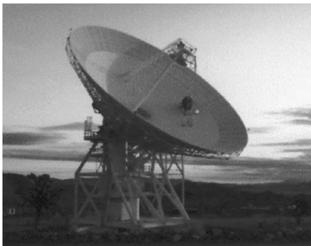
Figure 3. The 34-meter beam waveguide antenna at DSS 13. This figure can also be seen at the following website: http://deepspace.jpl.nasa.gov/technology/95_20/ant_5.htm . This figure is available in full color at http://www.mrw.interscience.wiley.com/esst .
