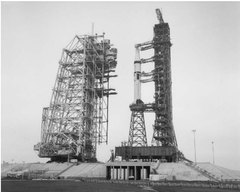
Figure 6. The Skylab vehicle on the “milk stool” on Pad 39B on 11 January 1971. The work stands on the Mobile Service Structure are clearly seen as it is propelled to the prelaunch position by the crawler (NASA photo). This figure is available in full color at http://www.mrw.interscience.wiley.com/esst .
