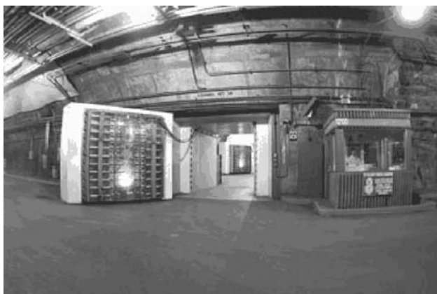
Figure 4. The Cheyenne Mountain Combat Operations Center (COC) is protected by a series of massive steel doors embedded in reinforced concrete located in a tunnel more than a thousand feet underground. Figure courtesy Cheyenne Mountain Operations Center. Picture can be found at http://www.cheyennemountain.af.mil . This figure is available in full color at http://www.mrw.interscience.wiley.com/esst .
