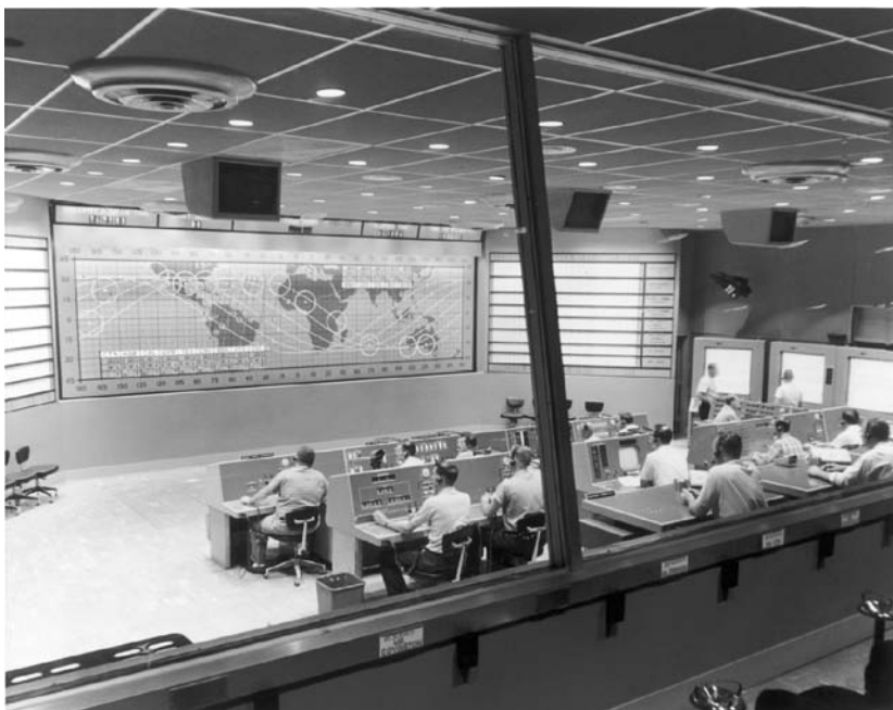
Figure 1. A reconstruction of the Mercury Control Center at Kennedy Space Center shows the world map with the ground tracks and station coverage (photo courtesy of NASA #KSC-62PC-128). This figure is available in full color at http://www.mrw.interscience.wiley.com/esst .
