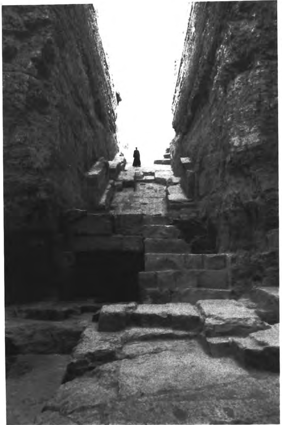
ABU ROWASH. The central section of the foundation level and the cleared descending ramp. (Photograph by M. Vallogia, 1997)
