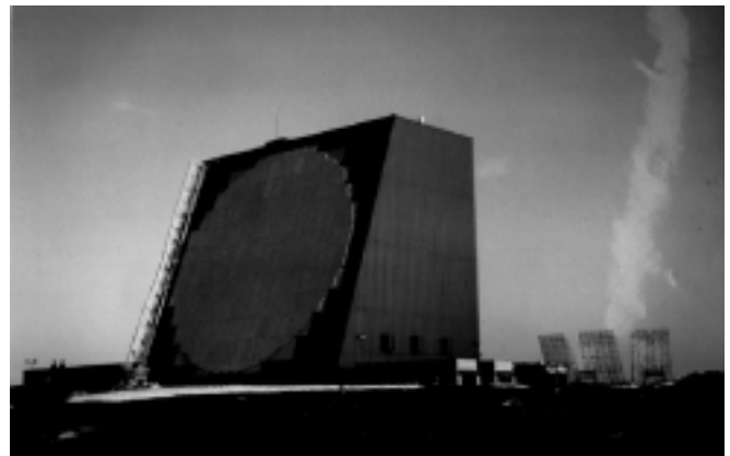
Figure R37 Cobra Dane phased array reentry instrumentation radar (Raytheon Co. photo).
