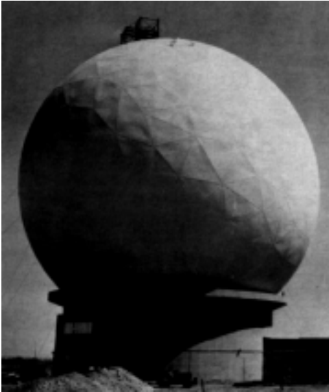
Figure R83 A 110-ft-diameter metal-space-frame radome (from Skolnik, 1970, Fig. 31, p. 14.26, reprinted by permission of McGraw-Hill).
