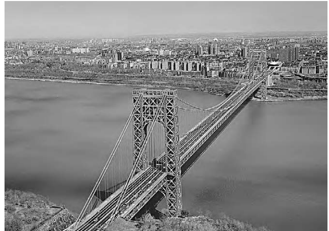
The George Washington Bridge, managed by the Port Authority of New York and New Jersey ( Library of Congress )
