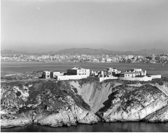
Fig. 40.20. Caroline Hospital on the Frioul Islands. The building is registered as a Historical Monument. In 1821, the government ordered the construction of the Berry Dike, joining Pomègues to Ratonneau, and the Caroline Hospital—a homage to Marie-Caroline de Bourbon-Sicile, princess of the Two Sicilies, wife of Duke de Berry—the creation was ordered from the architect M.-R. Penchaud. Used for the great epidemics of the nineteenth century for quarantine, the site was partially destroyed by the Allied bombings during the liberation of Marseille in August 1944. (a) An overall view of the Caroline Hospital. (b) In the background, Marseille. (c) The chapel, located at the center of the hospital complex (Moziconnacci photograph; courtesy of the Association Caroline, which operates the monument).
