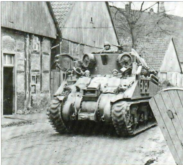
An M32 Tank Recovery Vehicle rolls through a village in north west Europe, 1945. Based on the M4 tank hull, these vehicles were used from 1943 onwards and used a fixed superstructure in place of the M4 turret. A large winch was fitted along with other special recovery gear and tools.
