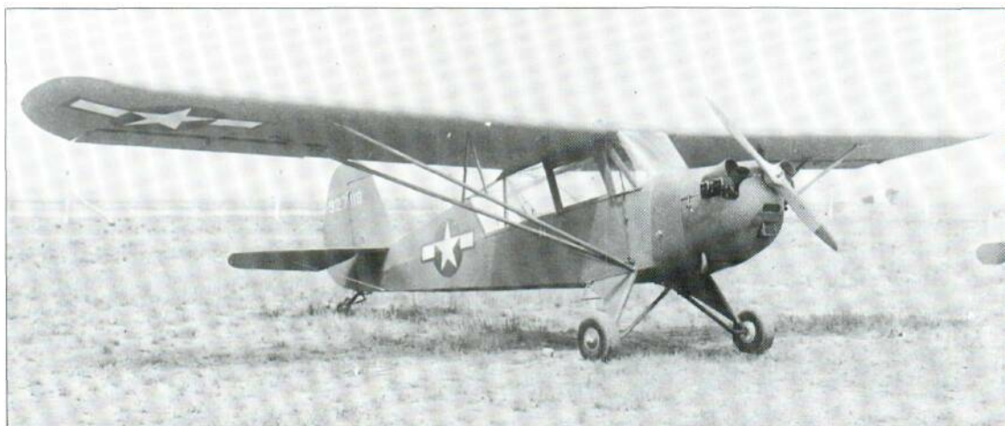
An Aeronca L-3C is seen during the last months of the war. Together with the Taylorcraft and Piper models of the Grasshopper, the L-3C was powered by a 65-hp O-170-3 Continental piston engine.
