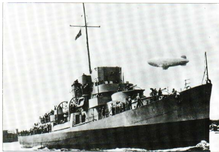
USS Harmon, a turbine-powered destroyer escort launched in July 1943, was named after a Navy Cross winner killed in the sea battle off Guadalcanal. The Harmon established a record, being delivered to the navy only 92 days after the keel was laid. Later vessels were built in even shorter times.
