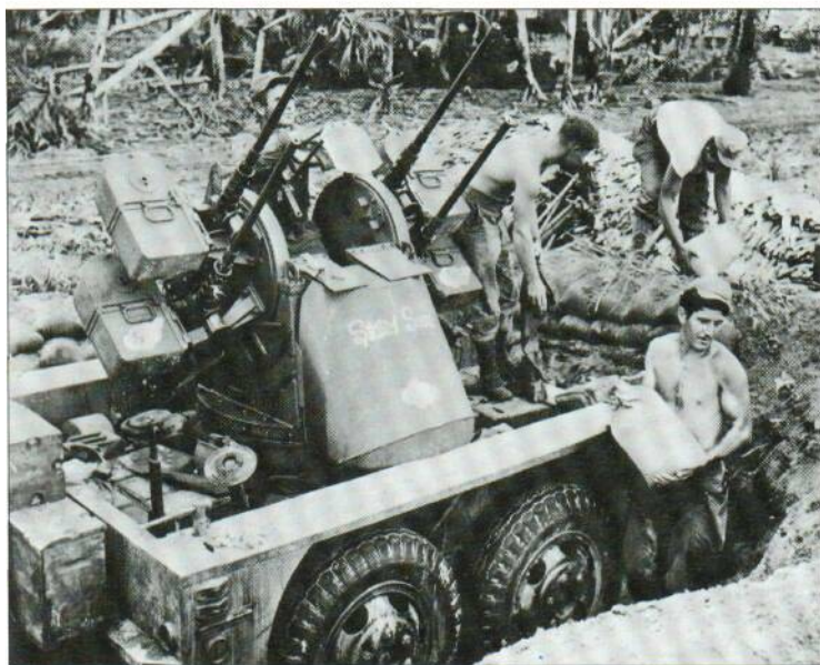
A Maxson mount is dug in in the Solomons. The gun layout can be clearly seen, as can the box magazines that held up to 200
