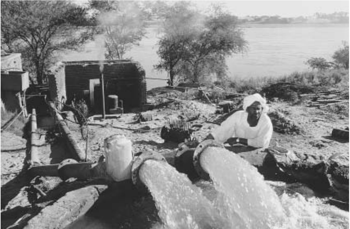
Water pipes carry water to irrigation ditches from pump stations located along the Nile River in Sudan. © Bojan Brecelij/Corbis. Reproduced by permission.
