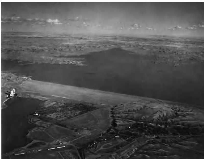
Fig. 12. Fort Peck Dam, Missouri River, Montana, the largest embankment dam by volume in the United States, 125,628,000 yd 3 (95,625,000 m 3 ). A hydraulic-fill dam, it was built between 1935 and 1939 for flood control, hydropower, irrigation, and navigation. (U.S. Army Corps of Engineers)
