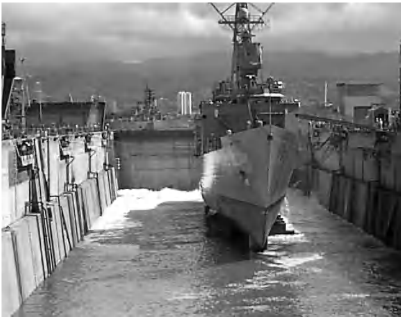
Fig. 6. Graving dock being flooded at Pearl Harbor Naval Shipyard. (U.S. Navy).
