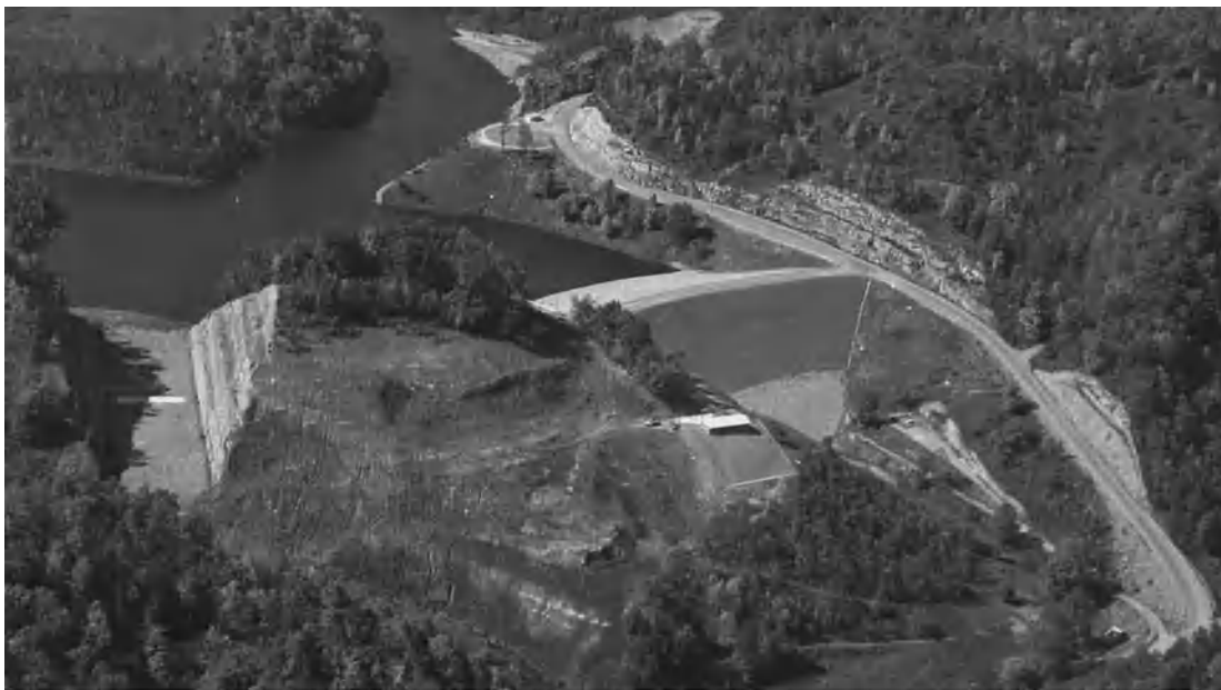
Fig. 5. Aerial view of North Fork Dam, a combination earth-and-rock embankment of the North Fork of Pound River, Virginia. The channel-type spillway (left center) has a simple overflow weir. (U.S. Army Corps of Engineers)
