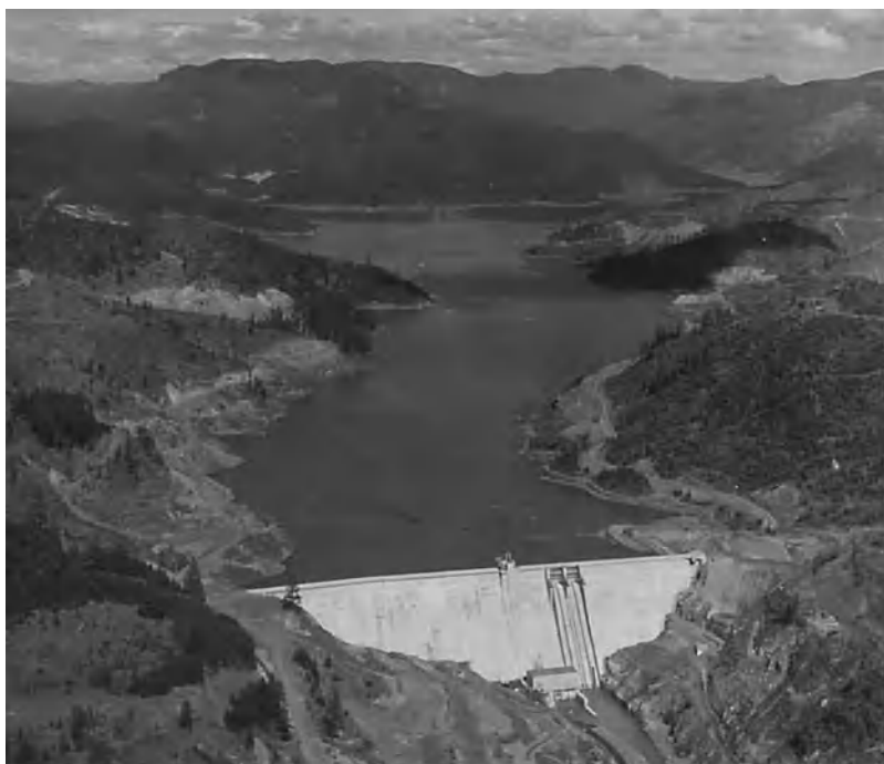
Fig. 7. Green Peter Dam, a concrete gravity type on the Middle Santian River, Willamette River Basin, Oregon. A gate-controlled overflow-type spillway is constructed through the crest of the dam; the powerhouse is at the downstream toe of the dam. (U.S. Army Corps of Engineers)
