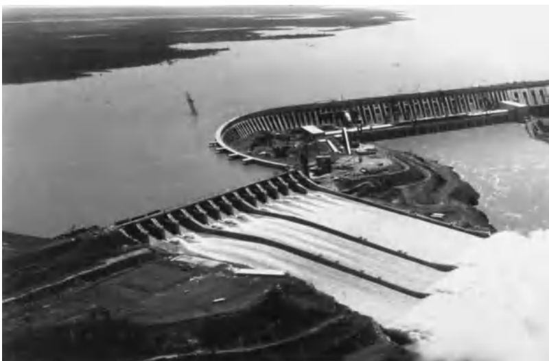
Fig. 4. Itaipu Dam, on the Paraná River between Brazil and Paraguay. An operating spillway with a flip bucket on the Paraguay side of the river is shown at left. The hollow concrete gravity dam with powerhouse construction at the downstream toe is shown at center. (G. S. Sarkaria, International Engineering Company, Inc.)
