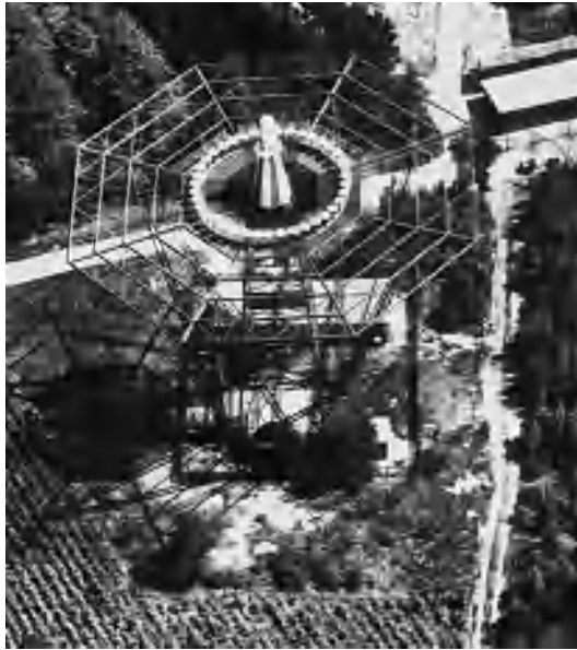
Fig. 1. Collocation of Doppler VOR and TACAN beacons installed on 100-foot high (30-m) tower with a counterpoise of 119-ft (36-m) diameter in forest near Frankfurt, Germany. Circular array consists of 39 loop antennas fed by solid-state commutator. Center carrier radiator is covered with plastic dome, which supports TACAN antenna.
