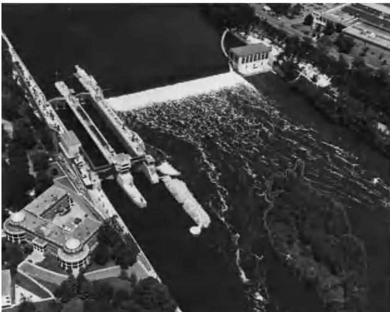
Fig. 2. Lock and Dam 1 on the Mississippi River between St. Paul and Minneapolis, Minnesota. Built in 1917 with a single lock to provide barge traffic to Minneapolis, the dam failed in 1929 and was rebuilt with twin locks in 1932. (U.S. Army Corps of Engineers)
