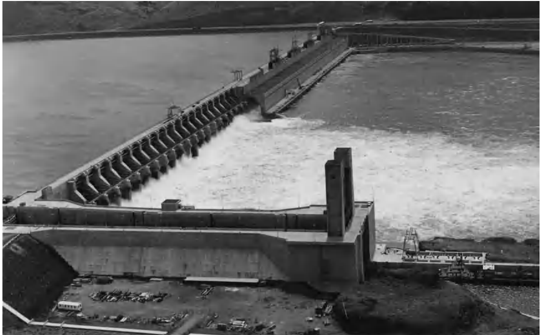
Fig. 1. John Day Lock and Dam, looking upstream across the Columbia River at Washington shore. In the foreground the navigation lock is seen, then the spillway beyond it, and then the powerhouse. The John Day multiple-purpose project has the highest single-lift navigation lock in the United States. (U.S. Army Corps of Engineers)
