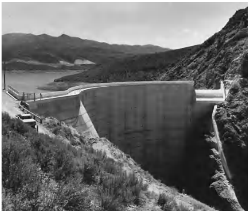
Fig. 10. East Canyon Dam, a thin-arch concrete structure on the East Canyon River, Utah. There is an uncontrolled overflow-type spillway through the crest of the dam at the right. (U.S. Bureau of Reclamation)
