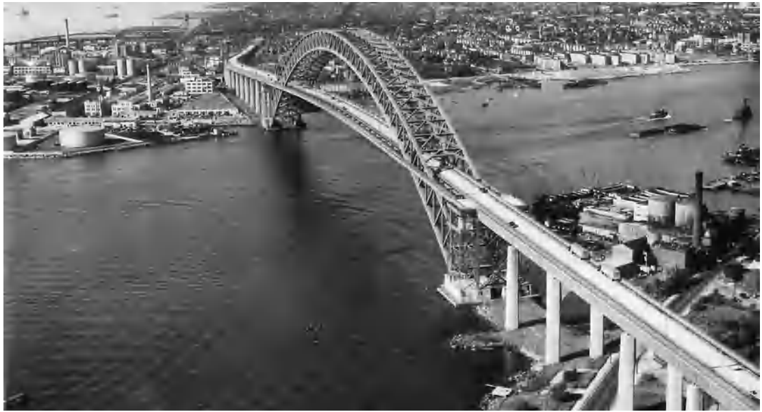
Fig. 4. Bayonne Bridge across the Kill Van Kull in New Jersey. (Port of New York Authority)
