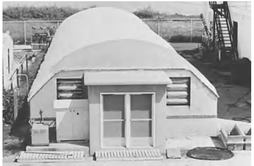
Fig. 5. Prototype inflated building housing raceways for intensive culture of marine shrimp. (National Marine Fisheries Service Laboratory, Galveston, Texas)
