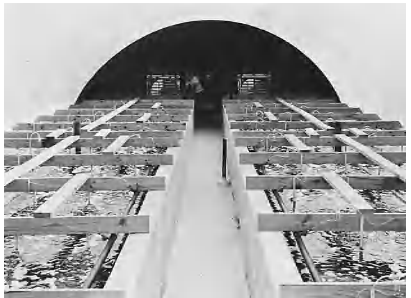
Fig. 6. Inside view of inflated building in Fig. 5 showing two long raceways used for shrimp production. (National Marine Fisheries Service Laboratory, Galveston, Texas)
