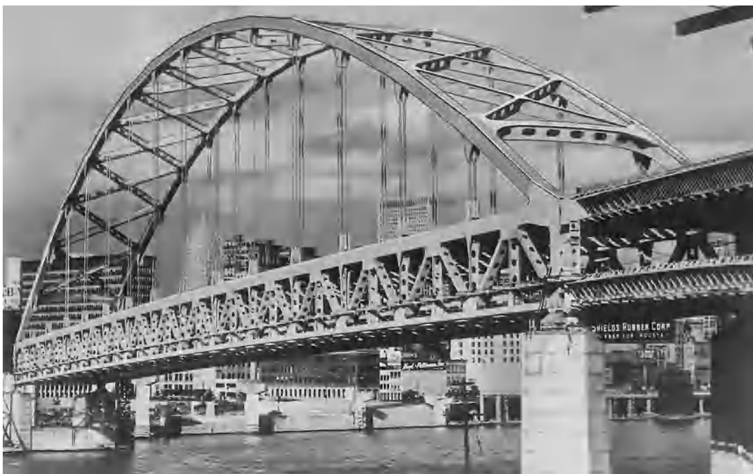
Fig. 3. Fort Pitt highway bridge, a double-deck tied-arch bridge across Monongahela River at Pittsburgh, Pennsylvania. Unusual are a truss instead of girders as ties, and box sections as arch ribs. (Lead Industries Ass.)
