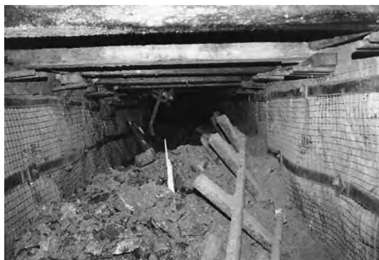
Rock burst damage to a mine opening from a small pillar burst. Note the track and rail heaved up almost 8 ft (2.5 m).
