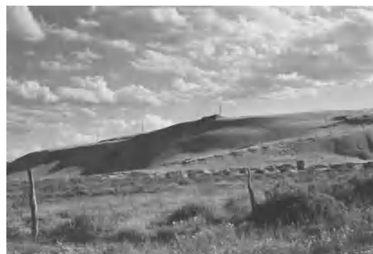
Fig. 4. Partial view of an operating mill tailings pile (Homestake Mining Company, Milan, New Mexico). The pile measures approximately 1000 m \times 1000 m (3000 ft \times 3000 ft), is 13 m (42 ft) high on average, and is entirely unprotected. In its 1.7 \times 10^7 m 3 ( 6 \times 10^8 ft 3 ), it contains 8000 Ci ( 2.9 \times 10^{14} Bq) of ^{226}\text{Ra} . The extracted uranium was enough to generate 100 GW(e)-year of electric energy in a reactor.
