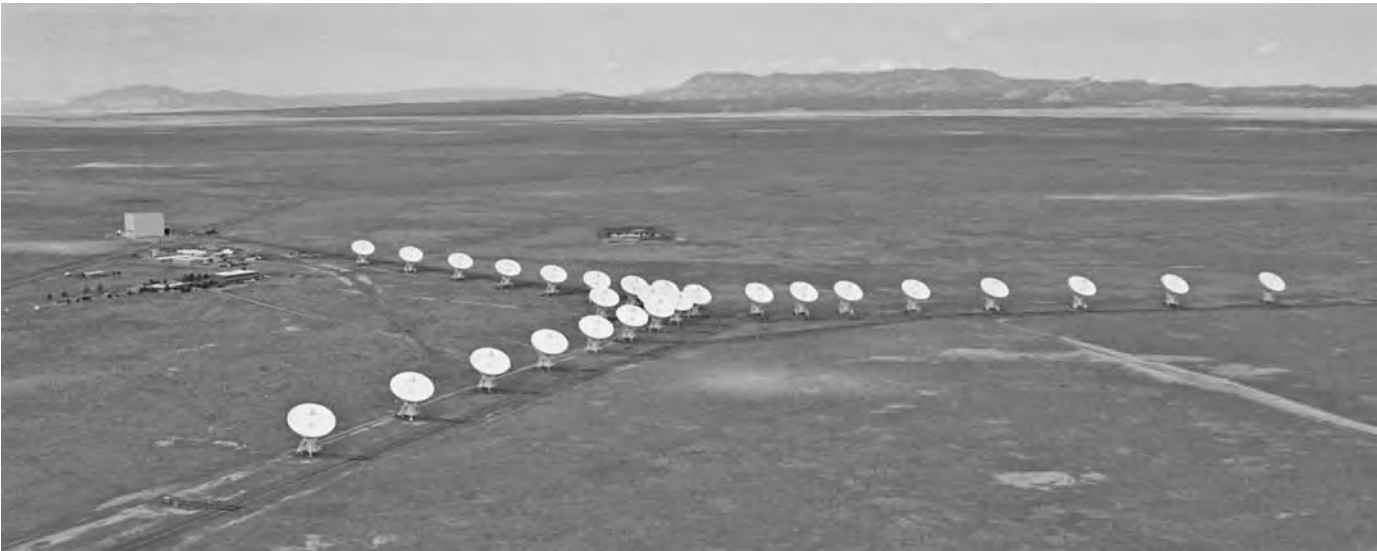
Fig. 3. NRAO 27-element Very Large Array near Socorro, New Mexico, in its most compact configuration. (NRAO/AUI/NSF)
