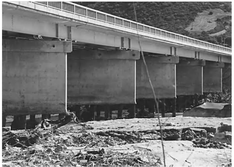
Fig. 3. River bed scour at a bridge crossing induced by sand mining in the river channel.
