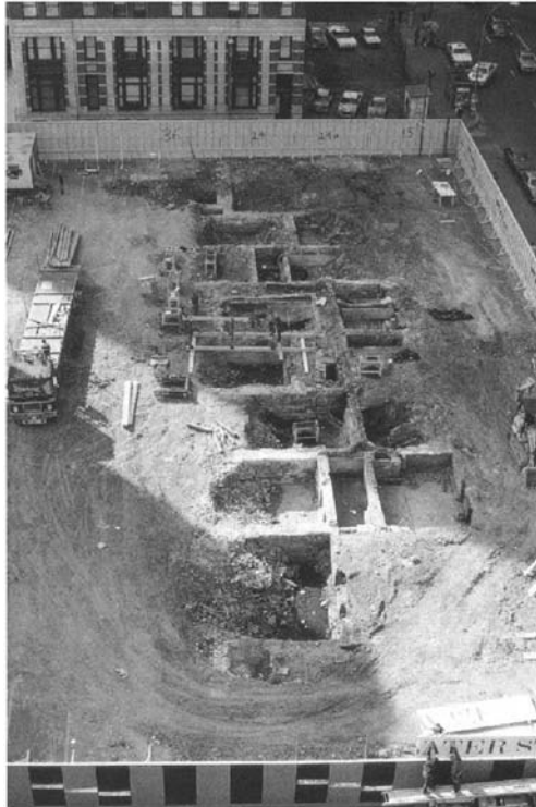
Figure 23 Excavation of 175 Water Street, New York City
