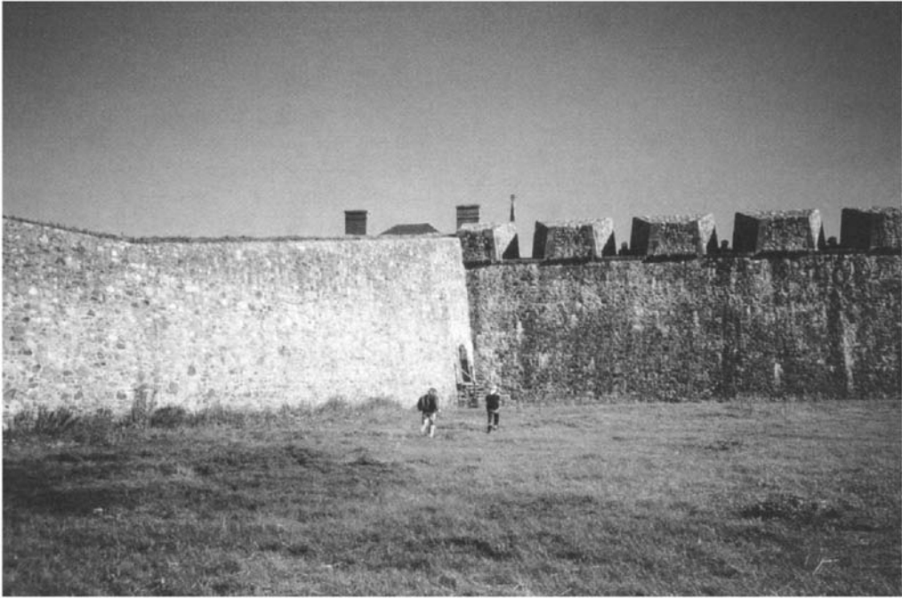
Figure 13 A section of reconstructed fortification wall at the Fortress of Louisbourg, Nova Scotia
