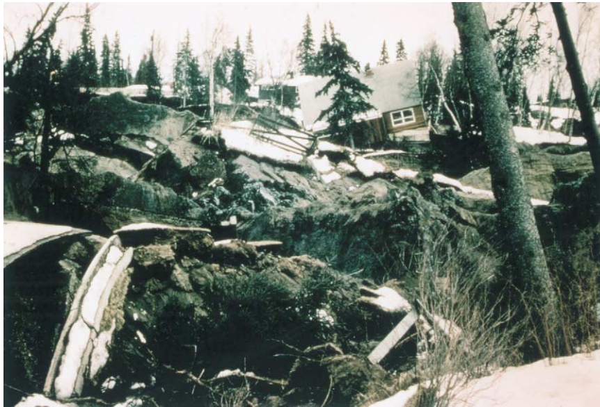
Figure 14 Destruction of the housing development at Turnagain Point above the Bootlegger Clay, Anchorage, 1994. The bluff moved 606 m towards the bay, and 75 homes were destroyed. Sand lenses in the clay lost strength (photograph National Geophysical Data Center, USA).
