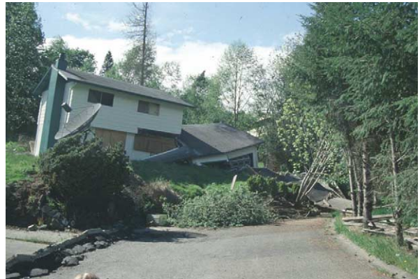
Figure 1 Home destroyed in 1998 in Kelso, Washington, by a thrust of soil under it as an ancient landslide reactivated, destroying 60 similar homes over a four-month period. Note the main street in the foreground has also been destroyed.
