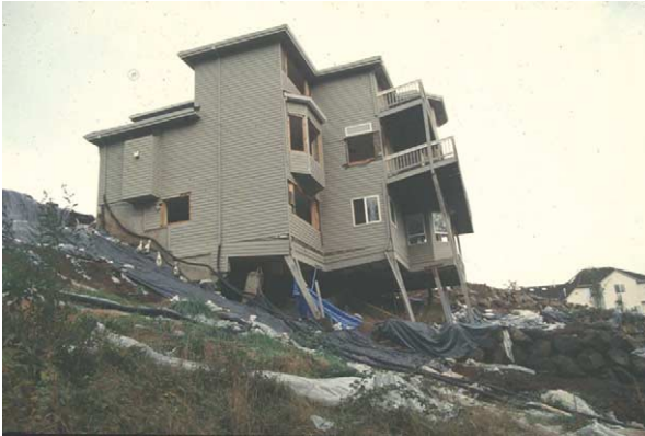
Figure 4 Slump destroys a house in Tigard, Oregon, USA; note deformation of supporting pillars. This home was built on the toe of an ancient landslide that reactivated in February 1996.
