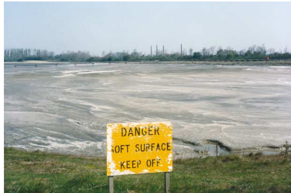
Figure 5 Lagoon filled with pulverized fuel ash.
