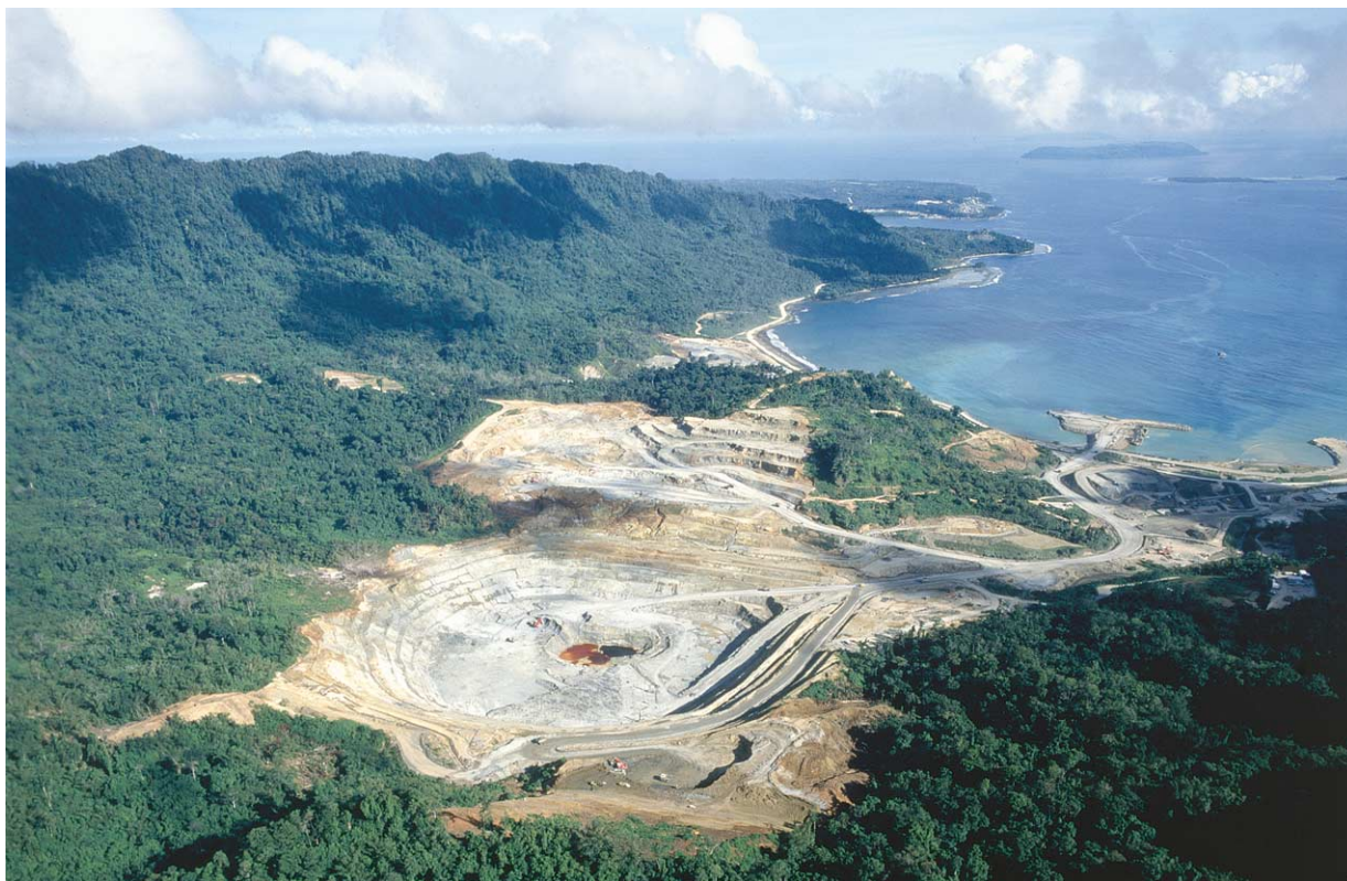
Figure 9 The open pit gold mine at Lihir Island, Papua New Guinea, under development in 1998, twenty months after inception of mining operations. The two pits, then about 40 m deep, and centred on ore bodies 1.5 km apart, will merge into a pit about 2 km across, with a planned depth of 300 m. The background and foreground hills are the walls of the volcanic caldera in which the epithermal gold-pyrite mineralization occurs. Photograph by courtesy of Rio Tinto PLC. Reproduced with permission from Evans AM (1995) Introduction to Mineral Exploration . Oxford: Blackwell p. 34.
