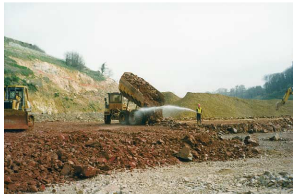
Figure 4 Watering rock fill during placement.
