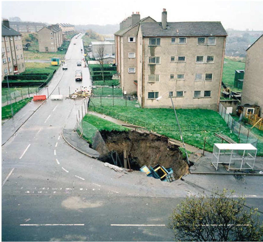
Figure 4 The result of a void migrating to the surface in old mine workings beneath a suburb of Glasgow. British Geological Survey photograph, in McCall GJH, de Mulder EFJ, and Marker BR (1996) Urban Geoscience . Rotterdam: Balkema.
