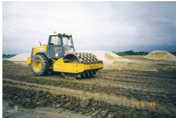
Figure 3 Compacting clay fill.
