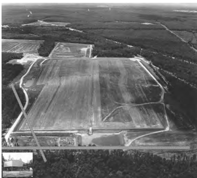
Figure 4. In situ gaseous nutrient injection system at the Savannah River Site 70-acre nonradioactive waste disposal facility depicting the 400 ft and 600 ft horizontal wells. Insert is gas-nutrient pumping station.
