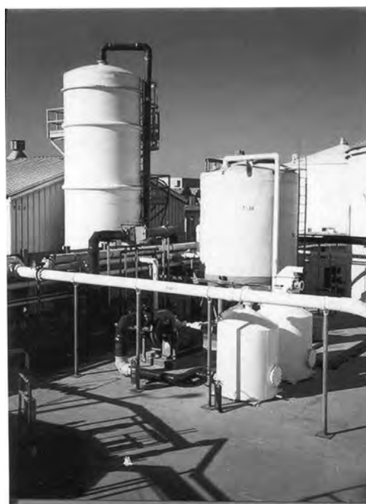
Figure 8. The North Island Naval Air Station biotrickling filter (Courtesy of Todd Webster, Envirogen Inc.).
