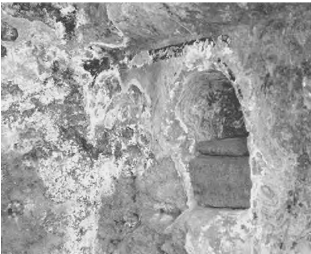
Figure 5. Salting on the surface of mortar in the tomb of Sevilha, Necropolis of Carmona, Spain. See color insert.
