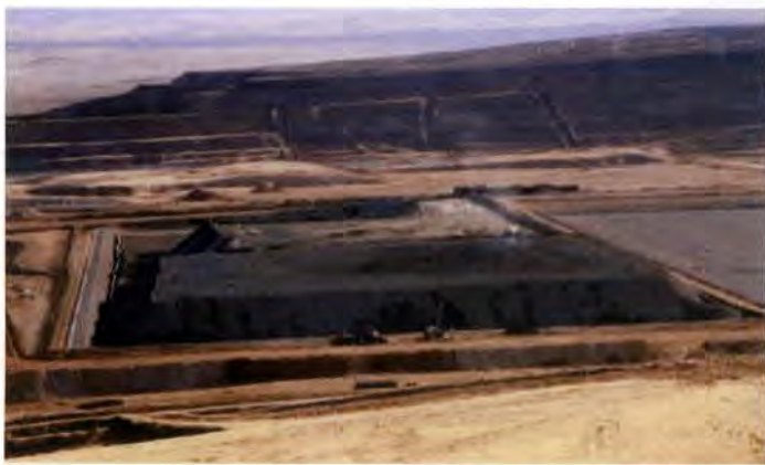
Bioremediation of Metals, Figure 6. One of the three biooxidation pre-treatment heaps measuring approximately 1,000 by 500 feet, with ore stacked to 30 feet, containing 709,000 tons of low-grade refractory ore. Courtesy of Dr. J. Brierley, Newmont Mining Corporation.
