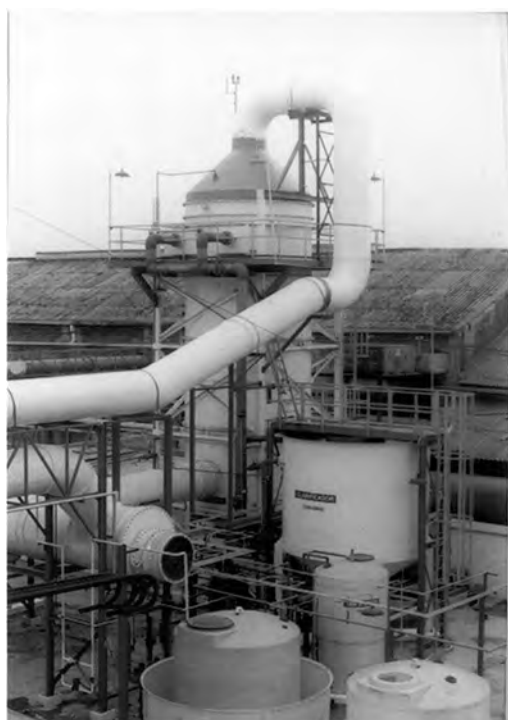
Figure 7. The Biocyd Celorey biotrickling filter (Courtesy of Mauricio Acosta Grupo Cydsa S. A. de C. V.).
