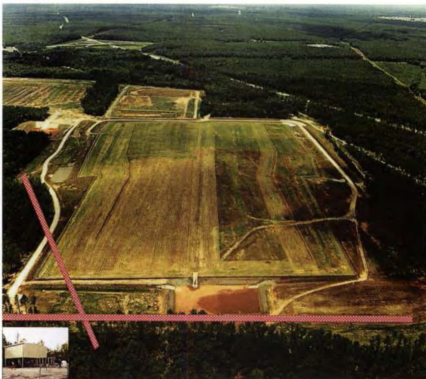
Methanotrophic Bacteria: Use in Bioremediation, Figure 4. In situ gaseous nutrient injection system at the Savannah River Site 70-acre nonradioactive waste disposal facility depicting the 400 ft and 600 ft horizontal wells. Insert is gas-nutrient pumping station.
