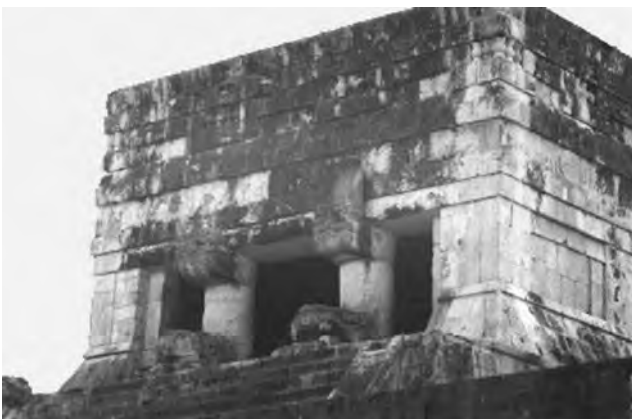
Figure 2. Mayan building in Chichen Itza, Mexico, showing blackening of limestone by epilithic and endolithic fungi and cyanobacteria. See color insert.
