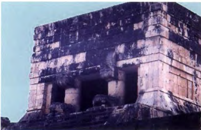
Biodeterioration of Mineral Materials, Figure 2. Mayan building in Chichen Itza, Mexico, showing blackening of limestone by epilithic and endolithic fungi and cyanobacteria.
