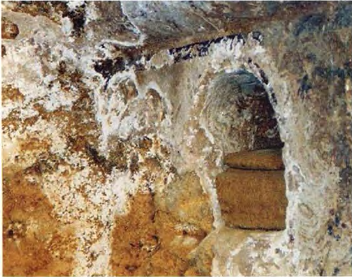
Biodeterioration of Mineral Materials, Figure 5. Salting on the surface of mortar in the tomb of Sevilha, Necropolis of Carmona, Spain.
