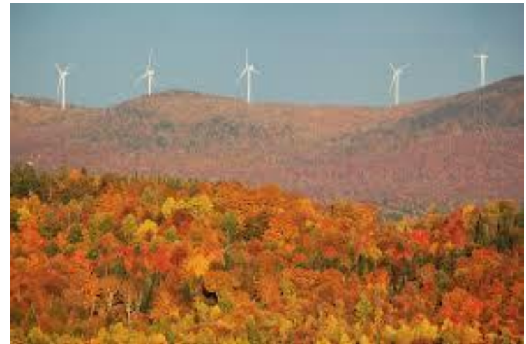
Lowell Mountain Wind Farm, Vermont
