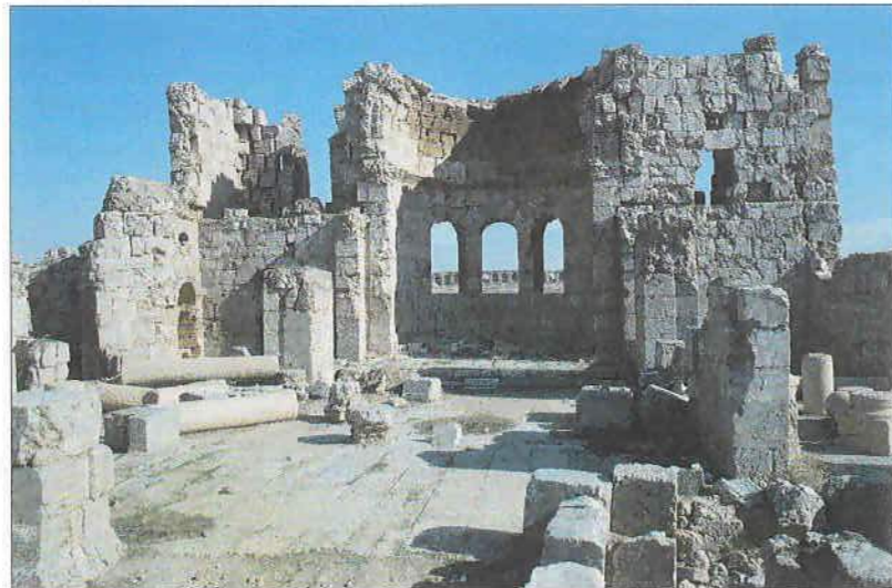
Right: the early 6th-century church of St Sergius and Bacchus at Rasafab, an important late Roman garrison town in Syria. The west end of the church was formed by a pair of towers; at the east end, the semi-circular apse was covered by a half dome.
