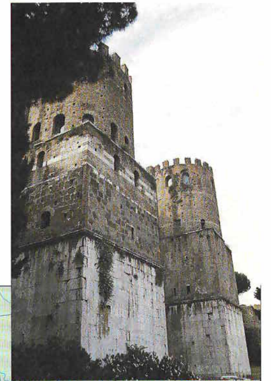
Above: the Porta Appia at Rome, now known as the Porta San Sebastiano, was originally built in the reign of Aurelian (270-75), but it and the walls on either side were heightened and strengthened first by Maxentius in the early 4th century, then again in 403 after the first Gothic invasion of Italy.
