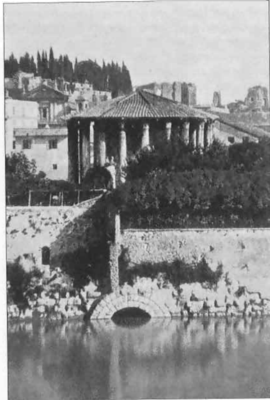
Above: the heart of Republican Rome, seen from the River Tiber. Opening into the river is the mouth of the Cloaca Maxima, the great sewer which drained the valleys between the hills of Rome, making possible the laying out of the Forum. Originally built by the Etruscans, it was substantially repaired during the reign of Augustus (27 BC–AD 14). Above it is the round temple of Hercules Victor, built in the late 2nd century BC.
