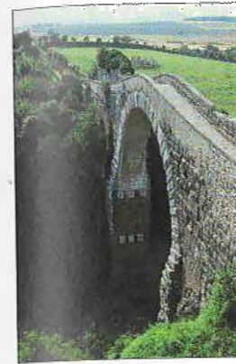
Above: it was the Etruscans who constructed the first major roads and bridges in central Italy. The road leading north from the Etruscan city of Vulci crossed the deep, narrow valley of the river Fiora on the Ponte della Badia. The original bridge consisted of stone piers supporting a wooden superstructure, but the latter was replaced by stone arches in around the 1st century BC.
