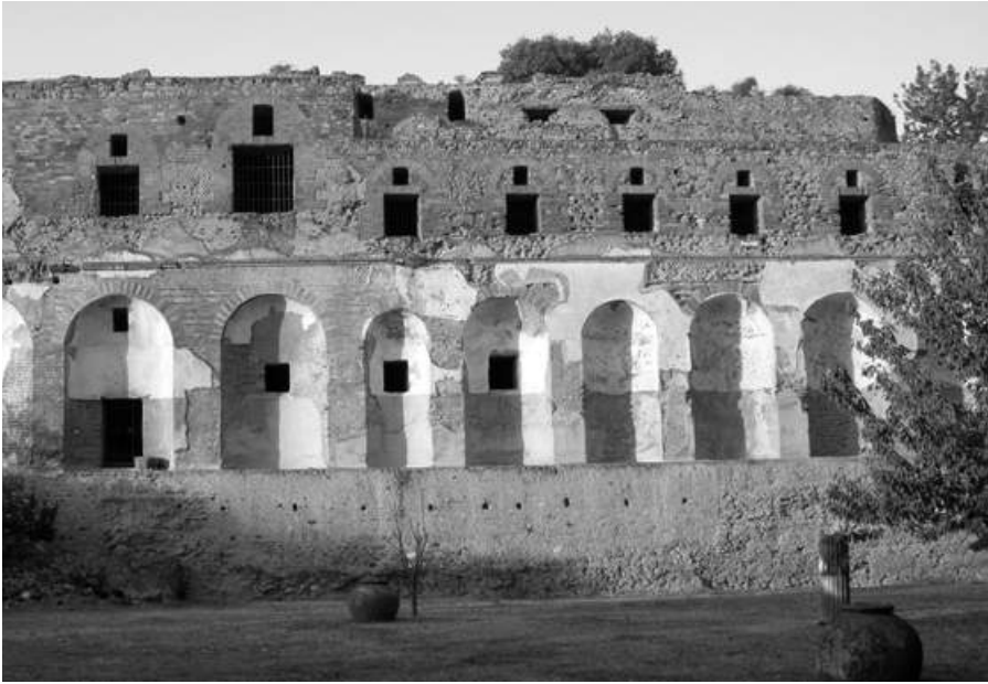
38. A bath block with a river view: the Sarno Baths. The bathing establishment was on the lower floors. Residential apartments occupied the upper levels.
