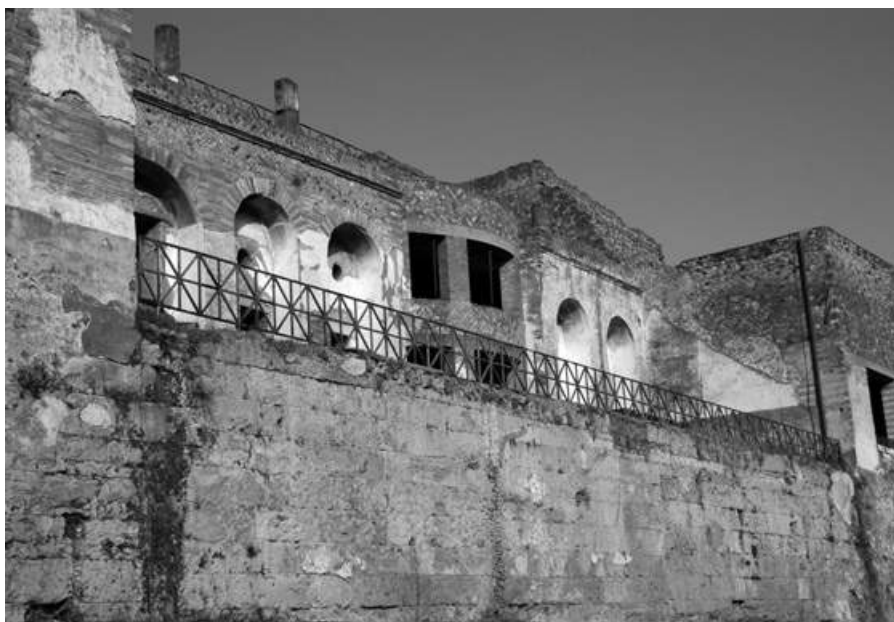
15. Located on the western edge of the city, above the old city wall, the House of Fabius Rufus enjoyed an enviable view over the sea. It was designed to make the most of this, with large windows and terraces.
