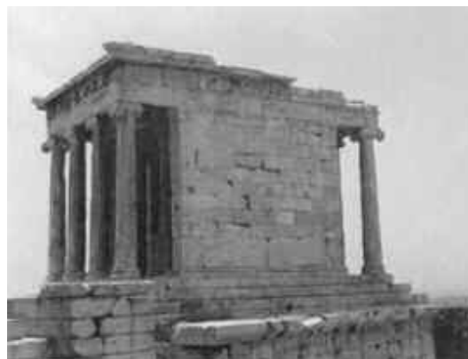
8.29 The Ionic marble temple of Athena Nike, constructed c. 425 BC. It has an almost square cella. The temple measures 17.75 × 26.75 ft (5.39 × 8.16 m). There are four prostyle columns at each end.
