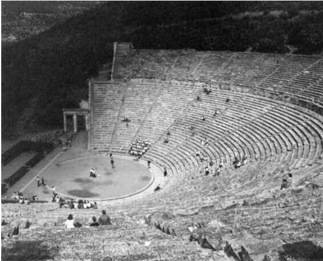
6.10 The theater at Epidauros was built in the later 4th century BC. It consisted of seating set in the hillside, a circular orchestra with doorways at each end of the parados, and (left) a skene, which was originally very tall.
