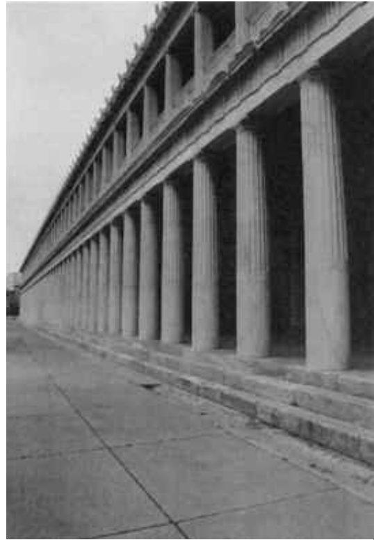
6.8 This imposing Hellenistic stoa at Athens defined the east of the agora. It was given to the city by Attalus II of Pergamum in the mid-2nd century BC. It had two floors with two aisles and rooms behind. Below are Doric columns; above, Ionic columns. It was restored by its American excavators.
