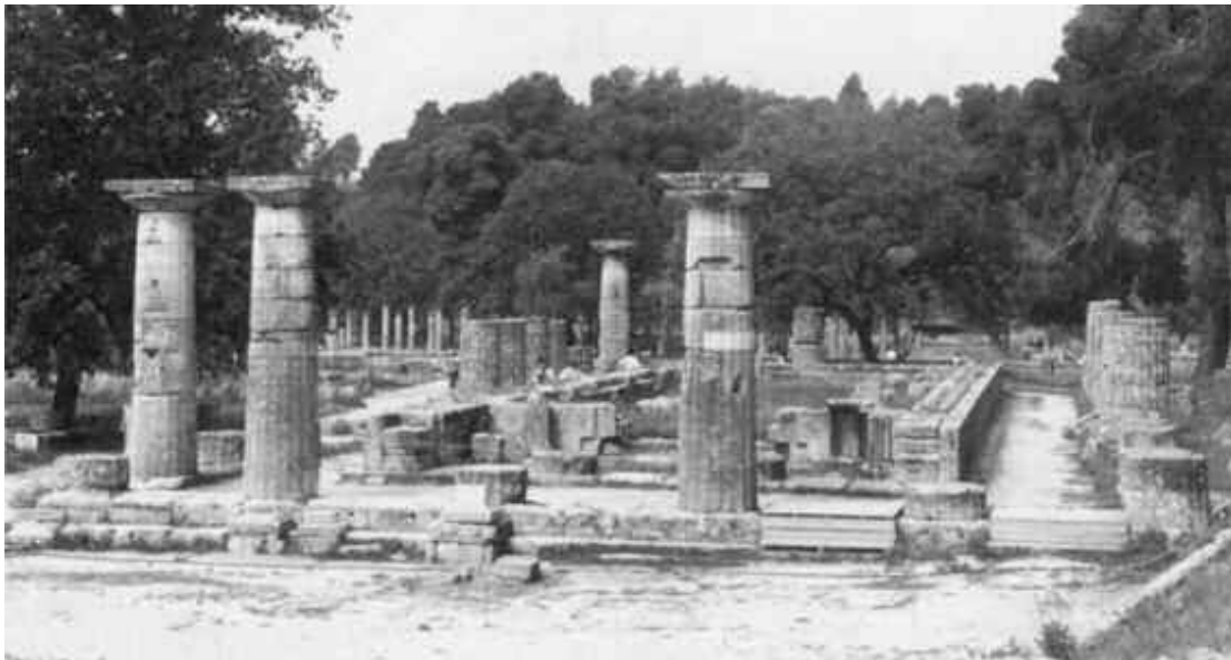
8.27 Archaic temple of Hera at Olympia. The cella walls were of limestone, and the upper part was of sun-dried bricks. The rest was of wood, apart from the tiled roof. The columns were replaced in stone from time to time.
