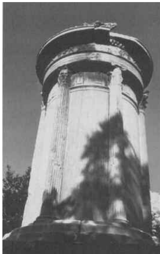
7.13 The Choregic Monument of Lysicrates at Athens, which stood in the Street of the Tripods. It originally supported a victory tripod won by Lysicrates who was the winning choregos in 335–334 BC. The monument consists of a square base and a tall cylinder with engaged Corinthian columns. The frieze has carvings of a narrative of Dionysus.
