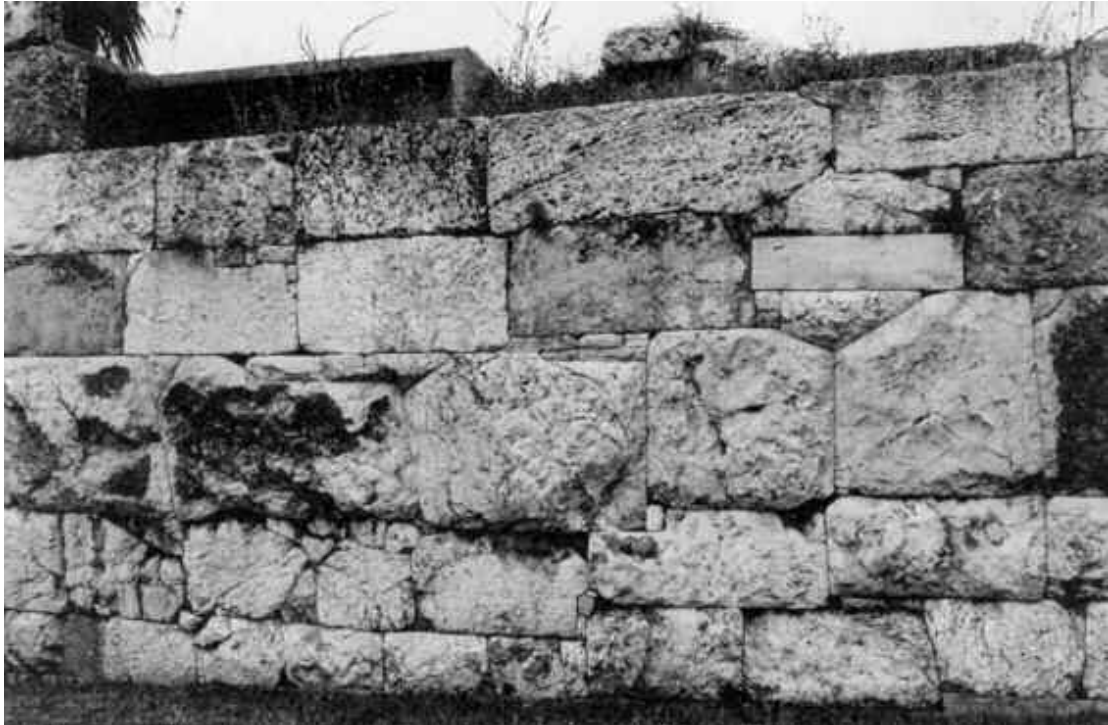
4.4 City walls near the Dipylon gate at Athens, where it passed through the Kerameikos cemetery. The wall was probably originally constructed in the time of Themistocles (the two visible lower courses are early 5th century BC), with rebuildings attributable to Conon (the polygonal masonry, early 4th century BC) and later (upper courses). Excavation of this stretch has shown it to be c.8 ft (2.5 m) wide; it was originally a stone wall with rubble infill, supporting a mud brick wall above.
