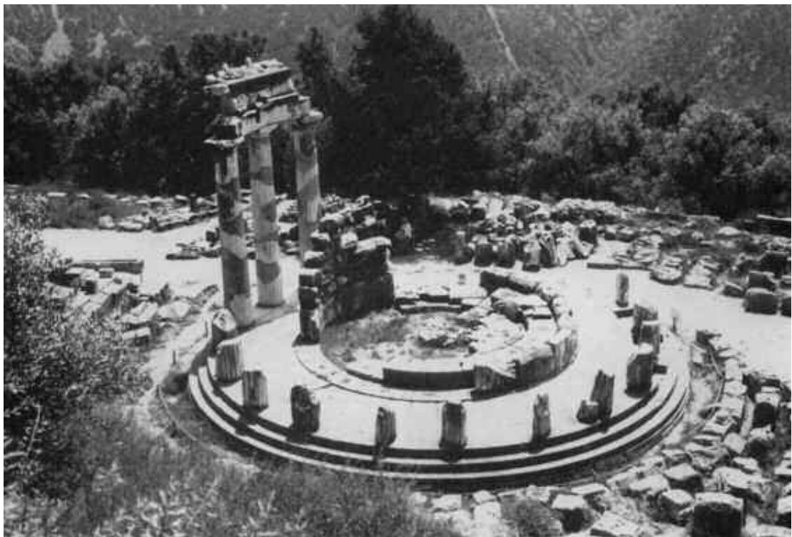
6.7 Tholos at Delphi of c. 375 BC. The architect may have been Theodorus of Phocaea, who apparently wrote a book on this tholos. There was an outer ring (pteron) of 20 Doric columns and an internal circular wall of a cella, with a ring of 10 adjoining Corinthian columns. The diameter of the entire building was 49 ft (13.5 m) and of the cella 28 ft (8.41 m). Its dedication and purpose are unknown.
