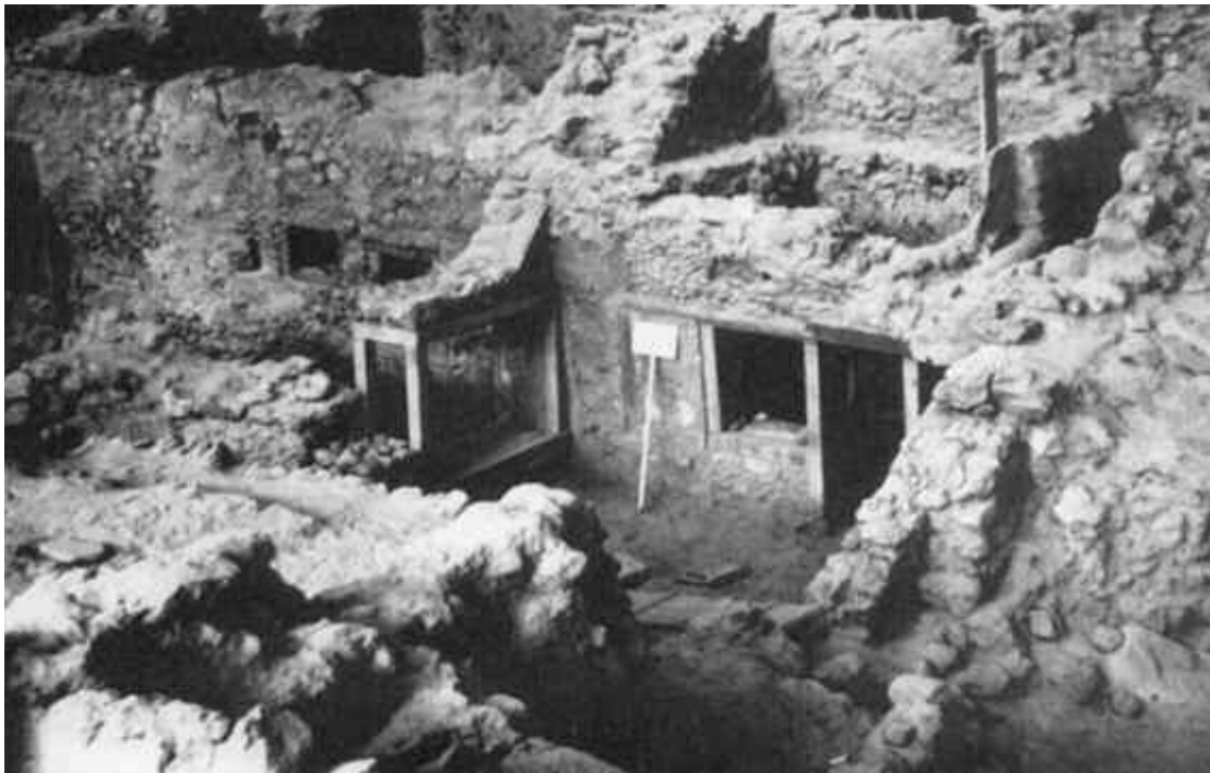
6.14 Middle Bronze Age houses well preserved by a volcanic eruption at the town of Akrotiri on Thera. They had up to three floors and were made of ashlar masonry, mud brick and timber-laced rubble, with evidence of doors, windows and wall paintings.
