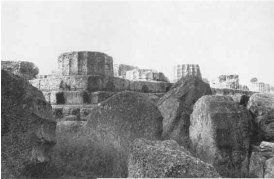
8.25 Early Classical Doric temple of Zeus at Olympia. It was begun c. 470 BC and was the work of local architect Libon of Elis. It measures 91 × 210.5 ft (27.68 × 64.12 m). In the foreground are collapsed column drums, from when the temple collapsed in a severe earthquake in the 6th century AD.
