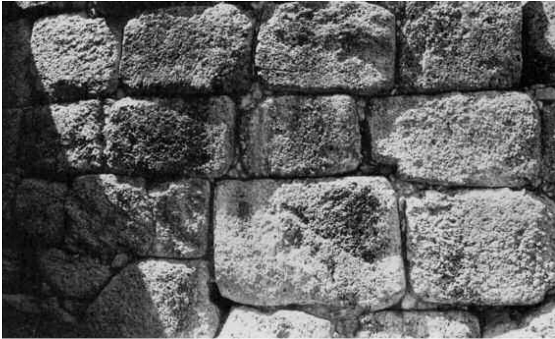
1.4 Cyclopean masonry outside the Lion Gate at Mycenae, dating to the late 13th century BC. These fortification walls were about 20 ft (6.09 m) thick.
