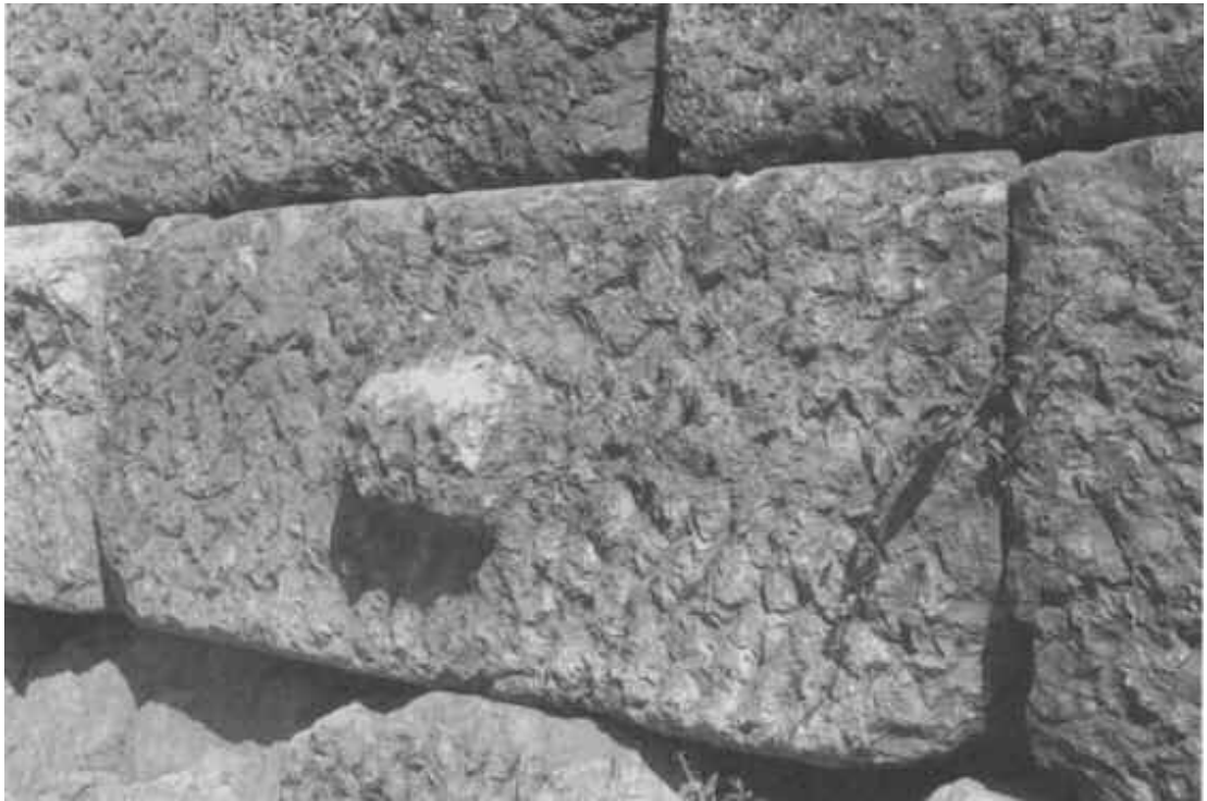
6.24 A lifting boss on a stone block on the Megarian Treasury at Delphi
