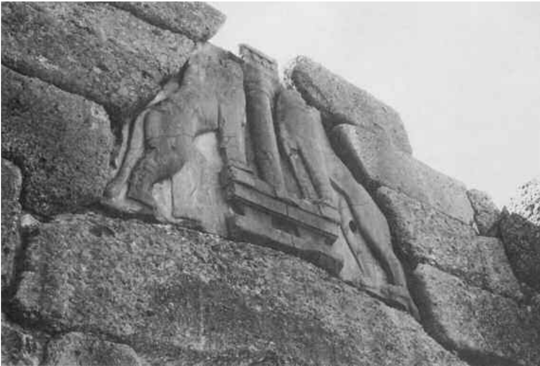
3.18 Lion Gate, Mycenae, c. 1250 BC. Over the gateway are massive slabs of stone and a supporting lintel. The lintel probably weighs about 20 tons. Above is a relieving triangle with a carved slab 2 ft (0.61 m) thick. It has a relief of two lions on either side of a column, but they have lost their heads.
